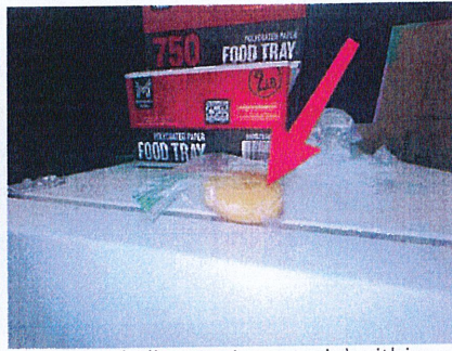
Discard all organic material within remediation area(s)
