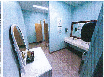
Women's Restroom 1 : perform small particle cleaning on exposed surfaces throughout entire area
