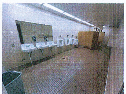
Men's Restroom 2 : perform small particle cleaning on exposed surfaces throughout entire area
