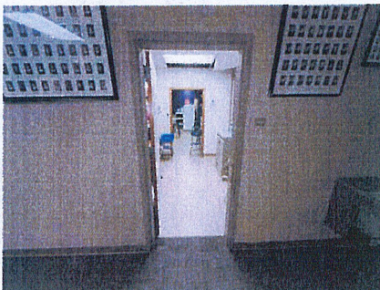
Storage 3 : perform small particle cleaning on exposed surfaces throughout entire area; porous contents with any visible growth should receive small particle cleaning or be discarded
