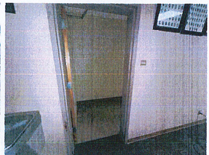
Women's Restroom 2 : perform small particle cleaning on exposed surfaces throughout entire area
