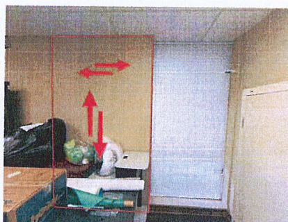
Classroom 15 : remove water/mold impacted drywall from floor to ceiling 2ft beyond any visible impact, clean all exposed framing
