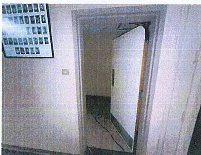
Men's Restroom 2 : perform small particle cleaning on exposed surfaces throughout entire area
