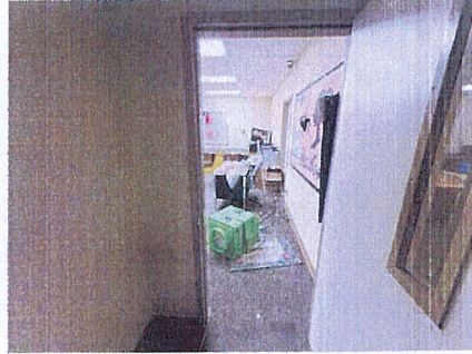
Computer Lab : perform small particle cleaning on exposed surfaces throughout entire area; porous contents with any visible growth should receive small particle cleaning or be discarded
