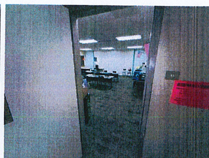
Classroom 13 : perform small particle cleaning on exposed surfaces throughout entire area, steam clean or remove all carpet; porous contents with any visible growth should receive small particle cleaning or be discarded
