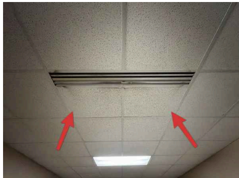
Ceiling Tiles : remove and replace all visibly impacted ceiling tiles throughout remediation areas
