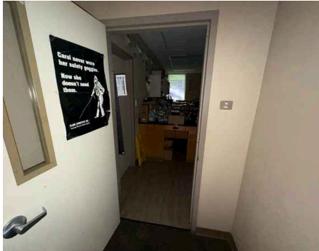
Classroom 16 : perform small particle cleaning on exposed surfaces throughout entire area; porous contents with any visible growth should receive small particle cleaning or be discarded
