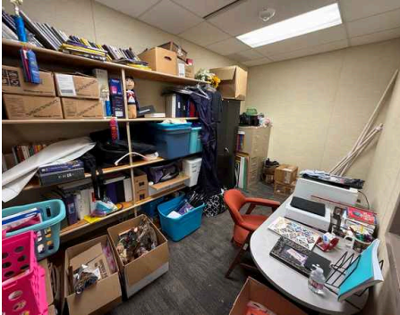
Classroom 6 Office : perform small particle cleaning on exposed surfaces throughout entire area, steam clean or remove all carpet; porous contents with any visible growth should receive small particle cleaning or be discarded
