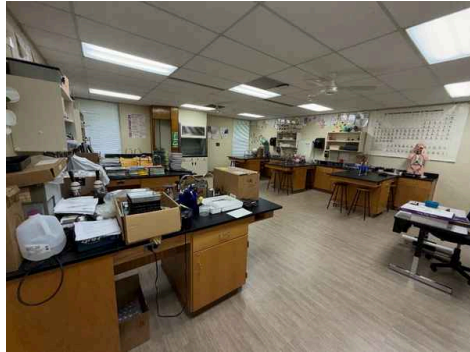
Classroom 16 : perform small particle cleaning on exposed surfaces throughout entire area; porous contents with any visible growth should receive small particle cleaning or be discarded
