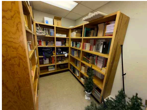
Storage 2 : perform small particle cleaning on exposed surfaces throughout entire area; porous contents with any visible growth should receive small particle cleaning or be discarded
