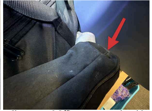
Classroom 6 Office : suspected mold growth observed
