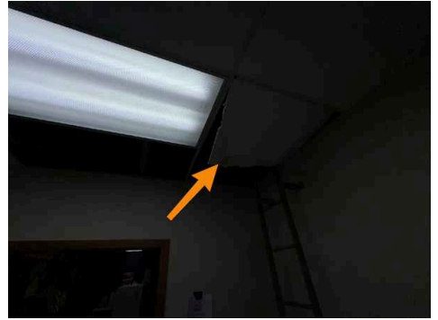
Storage 3 : water impacted material observed
