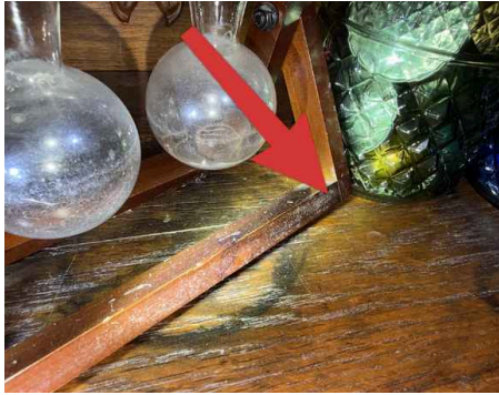
Office A : suspected mold growth observed
