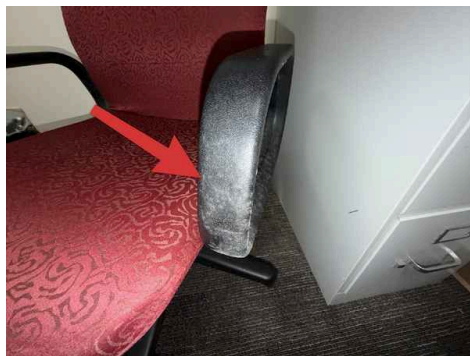
Office B : suspected mold growth observed
