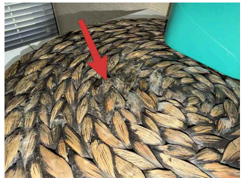
Classroom 4 : suspected mold growth observed
