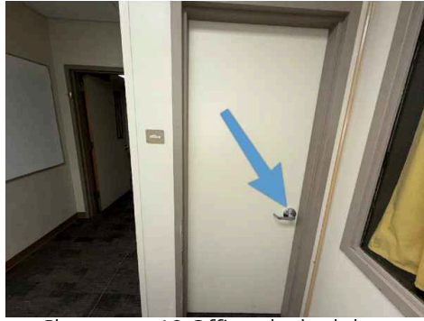
Classroom 10 Office : locked door
