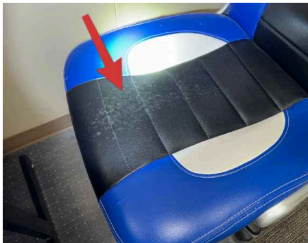
Classroom 7 : suspected mold growth observed
