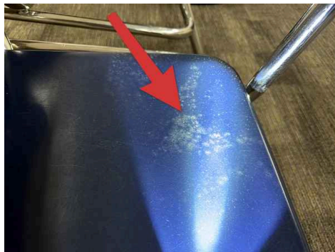
Classroom 4 : suspected mold growth observed
