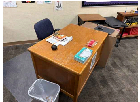
Classroom 3 : suspected mold growth observed
