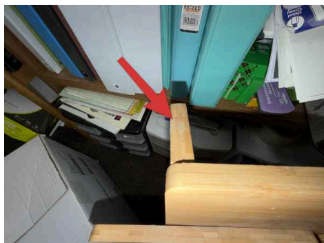
Classroom 12 : suspected mold growth observed
