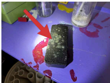
Classroom 6 : suspected mold growth observed
