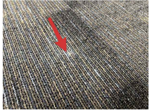
Classroom 5 : suspected mold growth observed
