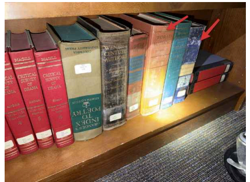
Library : suspected mold growth observed
