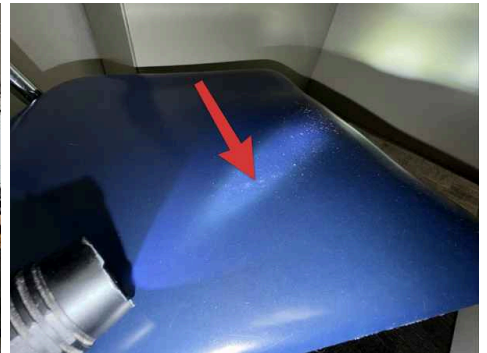
Classroom 8 : suspected mold growth observed
