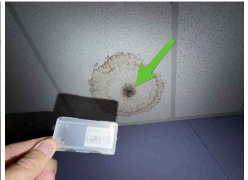
Library Work Room Ceiling Tile surface sample
